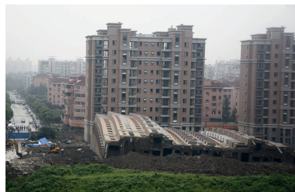
Figure 1: Collapsed apartment building due to unstable geological condition of the ground, and poor construction. Photo from Flickr, CC-BY-ND.
