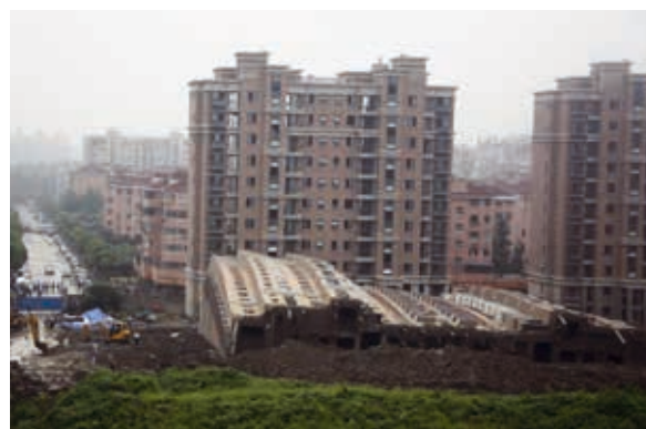
Figure 1: Collapsed apartment building due to unstable geological condition of the ground, and poor construction. Photo from Flickr, CC-BY-ND.
