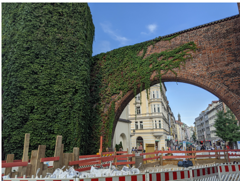
(a) Construction during summer
