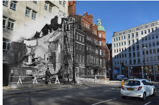
Figure 2.3.: London, destruction caused by the Nazi bomb attack; in the background London now with restored and new buildings [Eri16]
