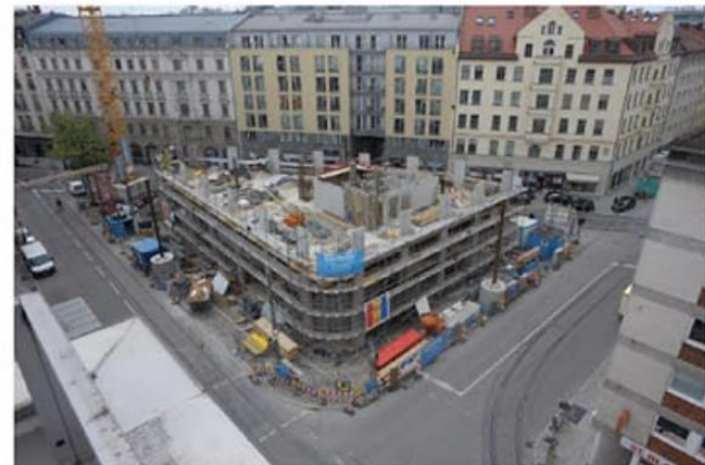
BIM Model and Construction Site [1]
