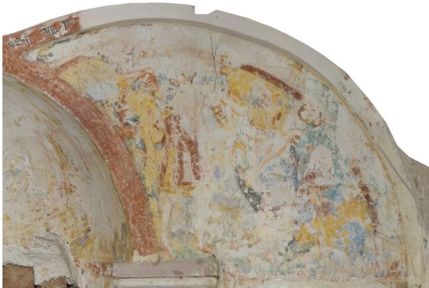
Detail of east wall. Arnold Kreisel, 09.04.2021.
