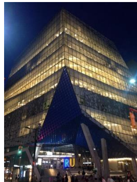
Ryerson Learning Center :
