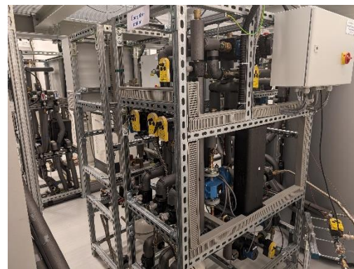
Figure 2: bidirectional heat transfer station in the CoSES laboratory
